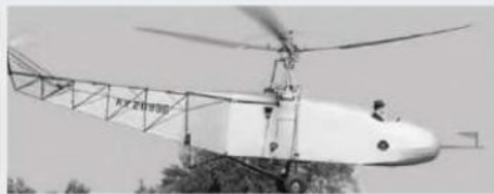
Igor Sikorsky's V-300 pioneered the single-rotor concept with cyclic and collective pitch for control and a tail rotor used for yaw.
